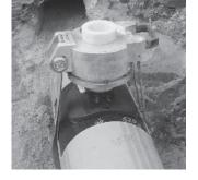
PE 100 SDR 11 Maximum permissible working pressure 16 bar (water) / 10 bar (gas)
